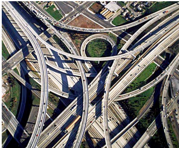
Complex service provision
